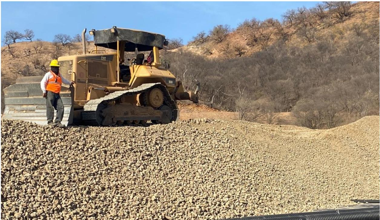
**Photo 4 – Heap leach pad loading**
